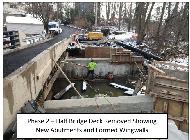
Bridge C-09, Single-Lane, Self-Yielding Traffic Pattern – Phase 2
